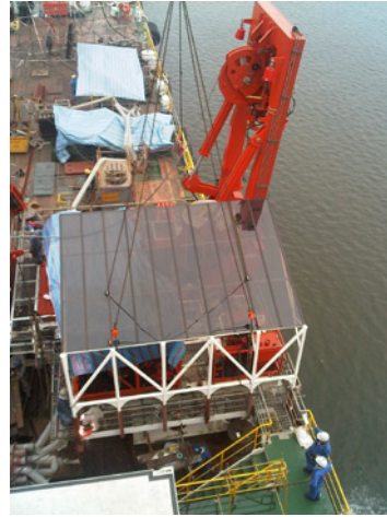
☛ Installation of Submarine roof
